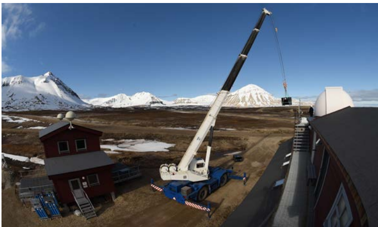
Fig. 3: The radar attached to the hook. (René Bürgi)
